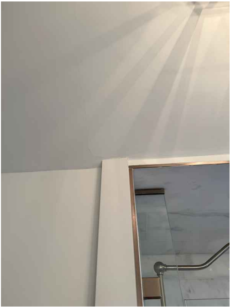
2nd Floor Bathroom
