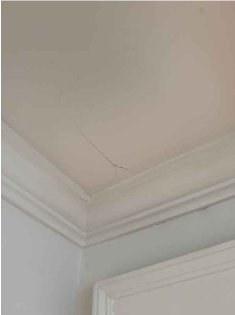
Kitchen to Dining Room Hallway
