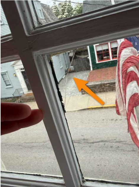
2nd Floor Hallway
