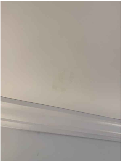
2nd Floor Bathroom
