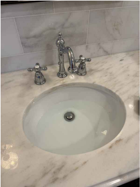
2nd Floor Bedroom Bathroom
