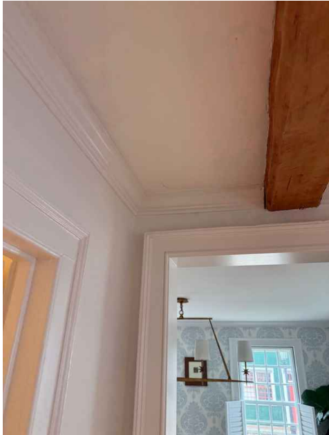
Kitchen to Dining Room Hallway
