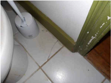
1st Floor Bathroom
