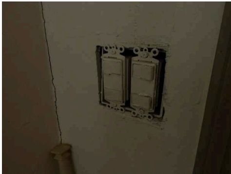
Unit 57 2nd Floor Bathroom
